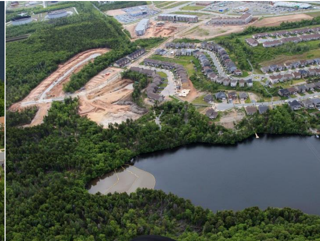
South end of Russell Lake, looking West South-West, showing siltation booms
