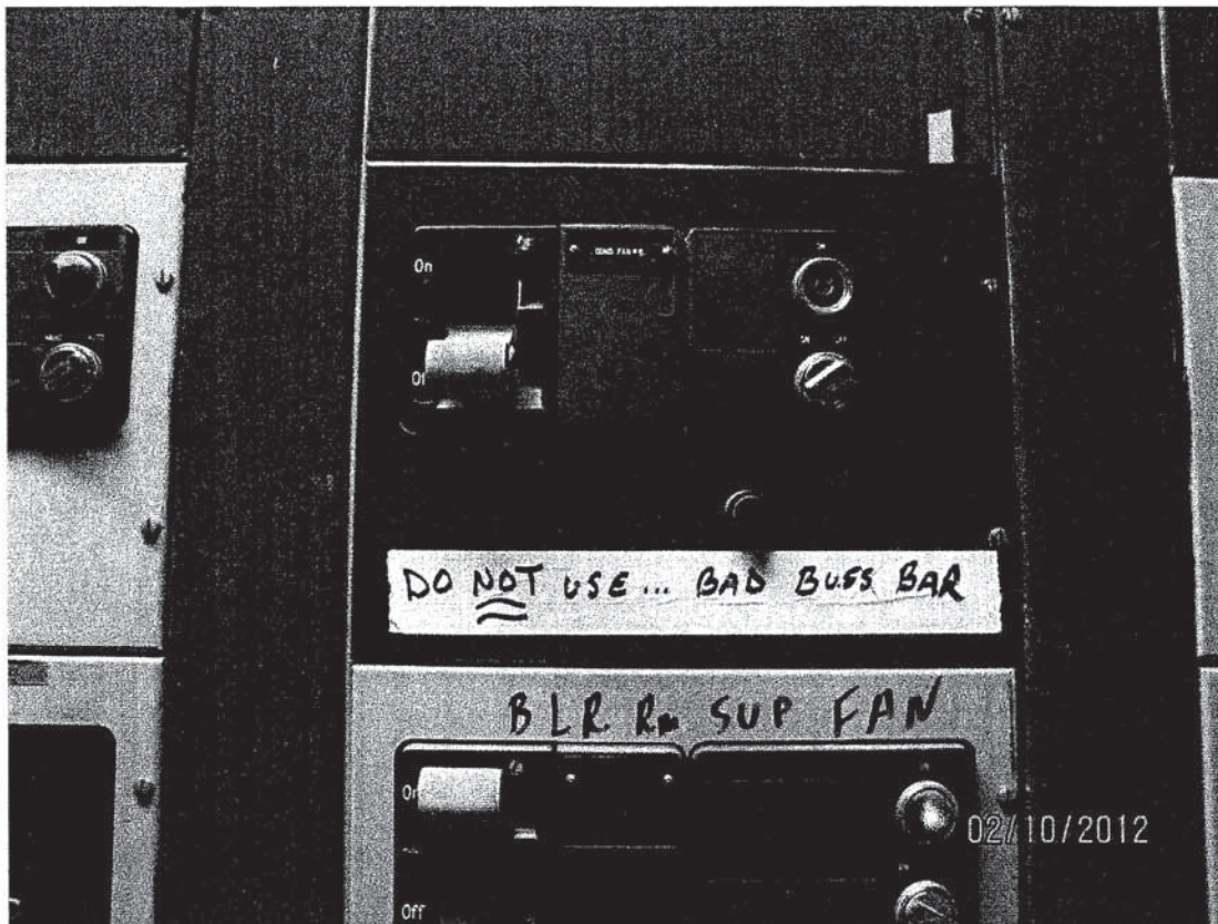
Main MCC Cabinet – HMC Engine Room
