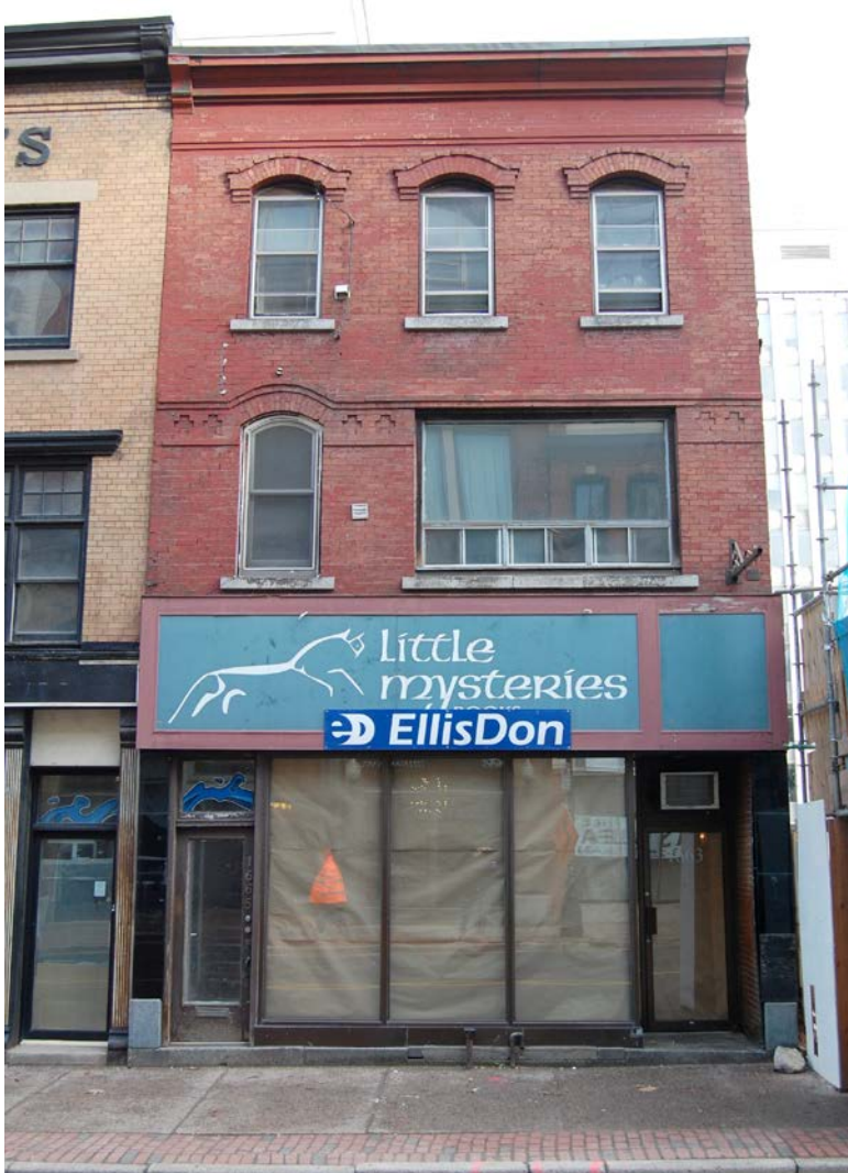
Existing façade along Barrington Street
