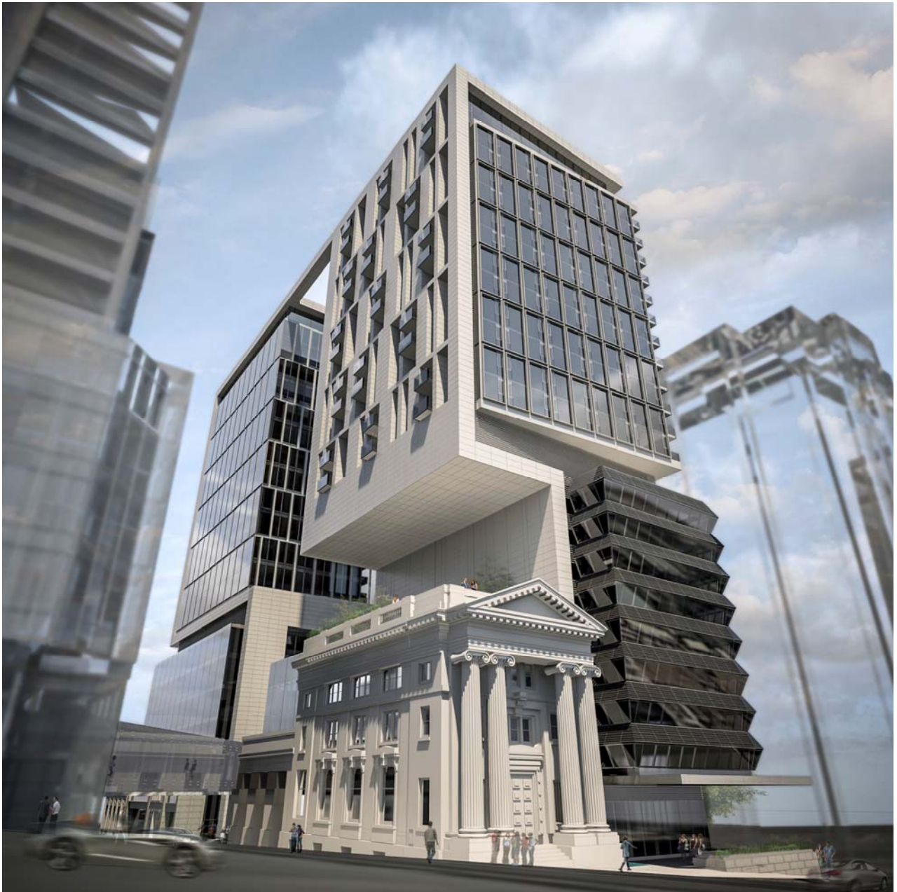
View of South facing elevation from George Street.
