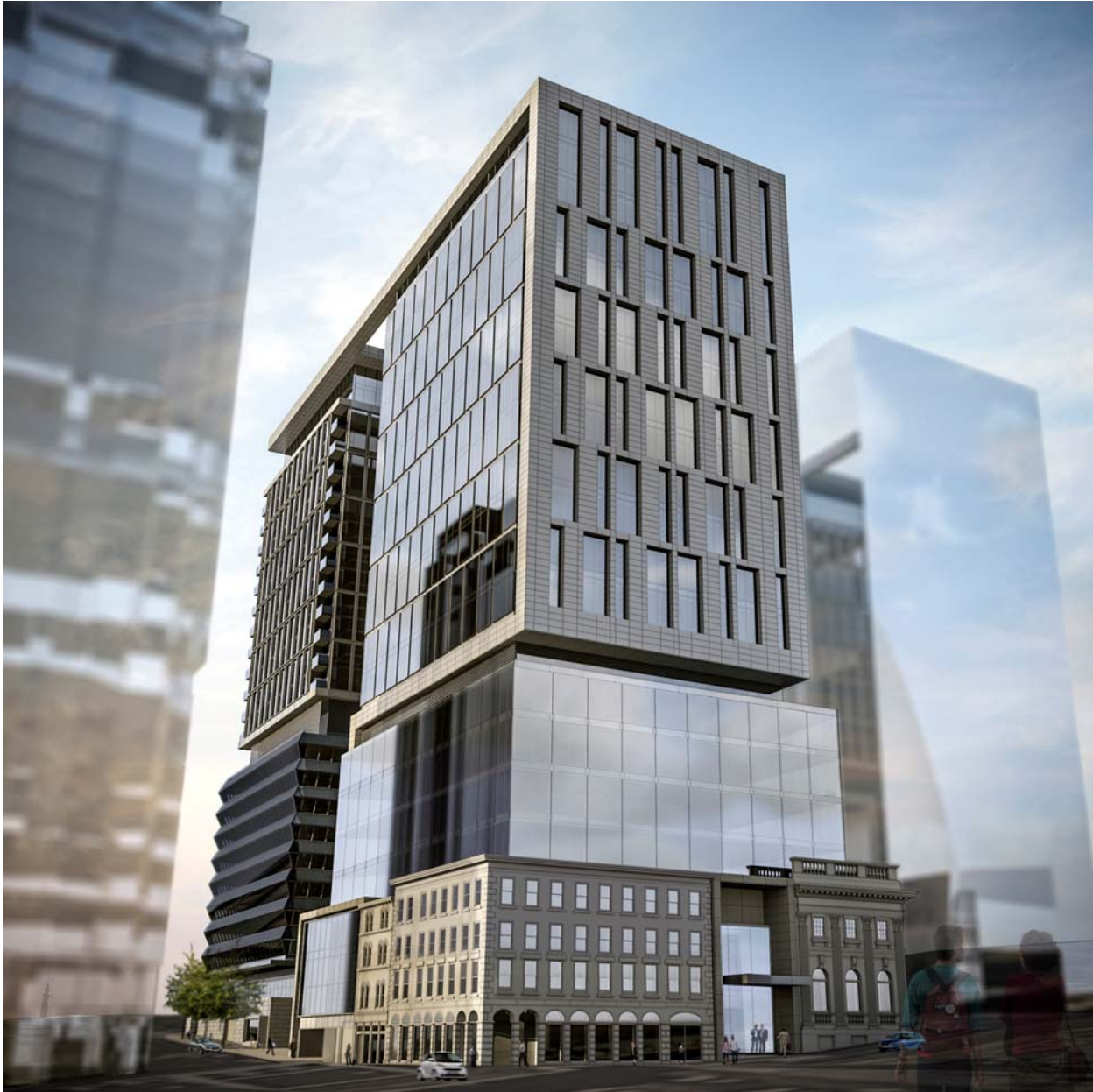
View of North facing façade along Hollis Street.
