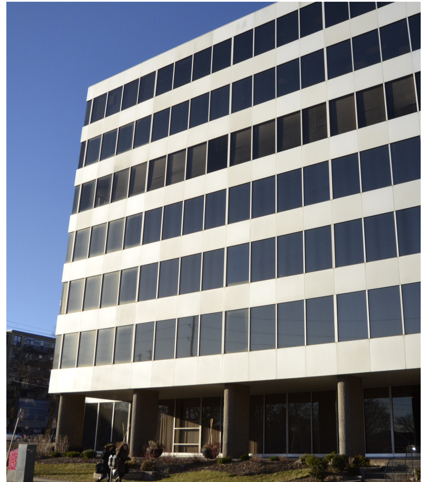
Existing Building 5151 Terminal Road Photograph
