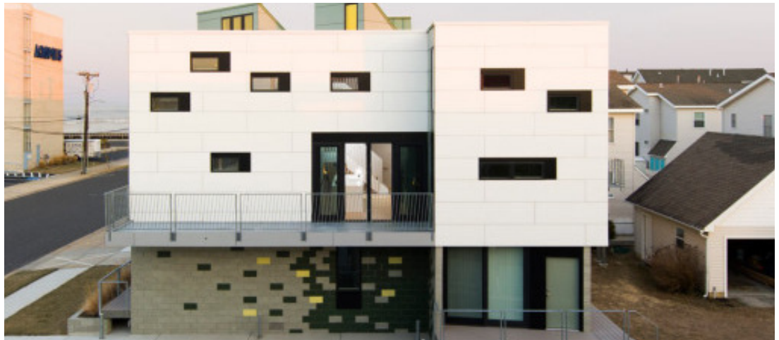
Example of white high pressure laminate rain-screen paneling system
