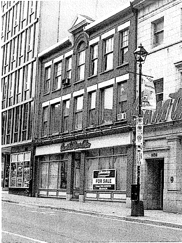
1652 Barrington St - Harrison Building
