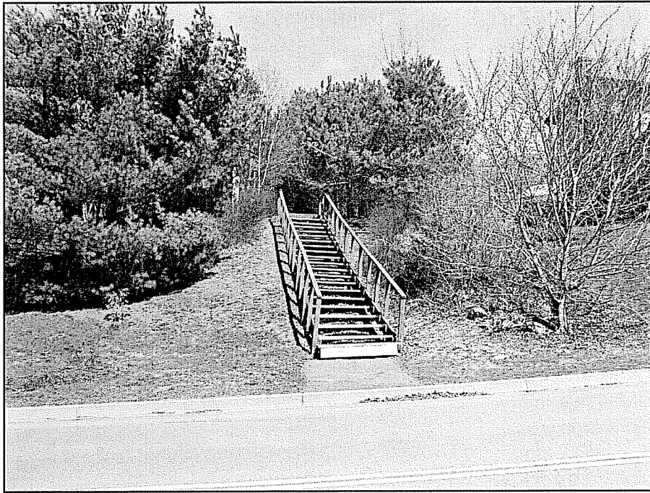
Figure1: Entrance to Golf Links Park from Peregrine Crescent.
