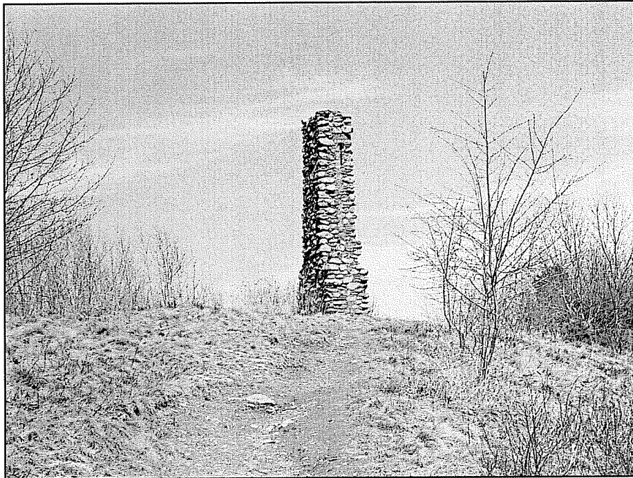
Figure 4: View from the footpath to the Chimney.
