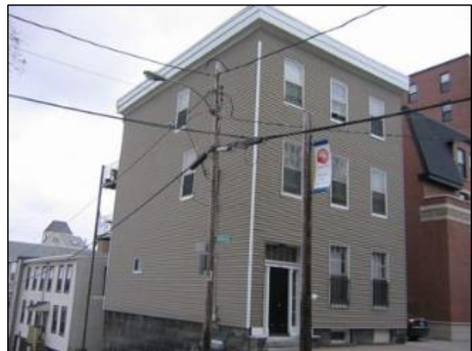
Figure 7: based on photographic evidence (Figure 6), a financial incentives program could support a restoration project to return the brick cladding and lintels on the second storey of this Italianate building on Hollis Street
