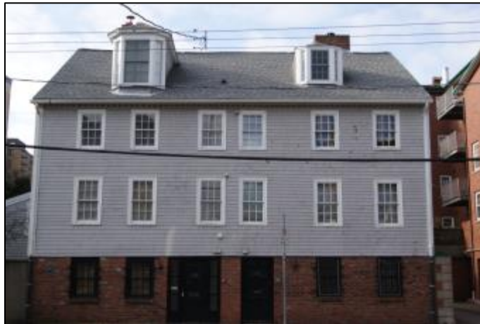
Figure 2: one of the older buildings in the Old South Suburb, constructed between 1796 and 1805, the Alexander McLean House is a good example of the Georgian style of architecture with two central entrances, three-bays wide, and it is deep from front to back.
