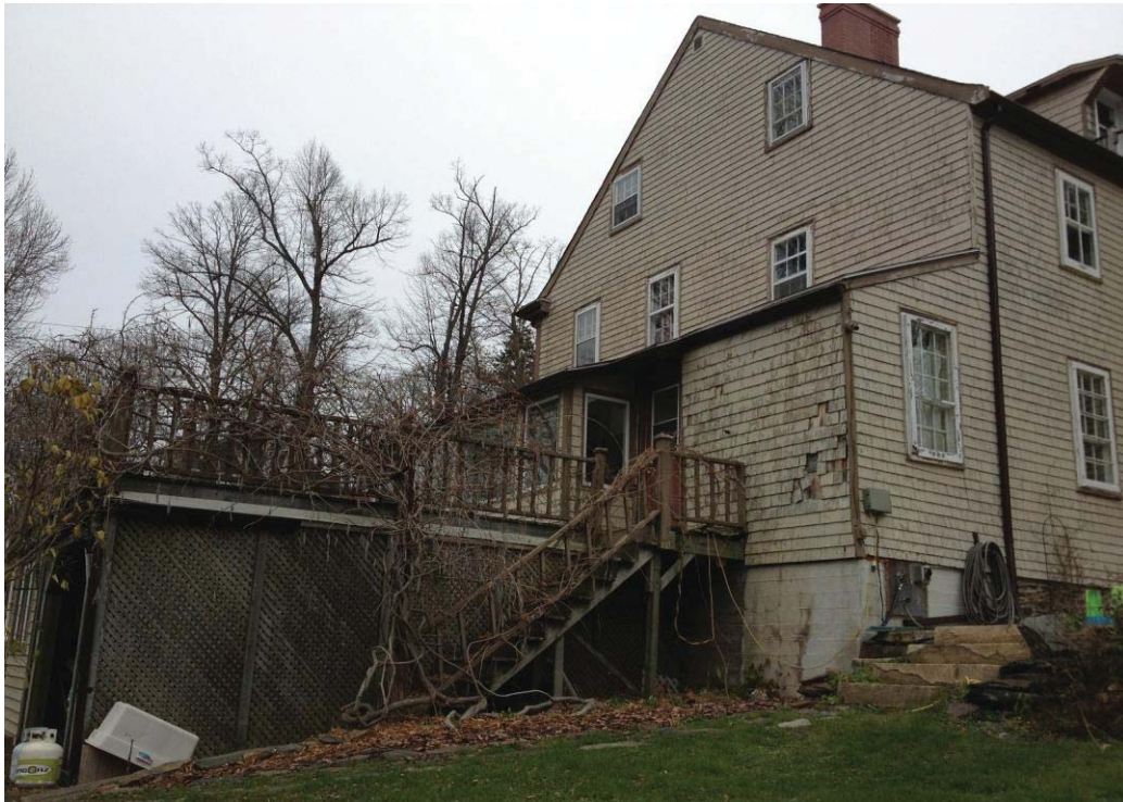
Photograph 3: Rear view of sunroom and carport
