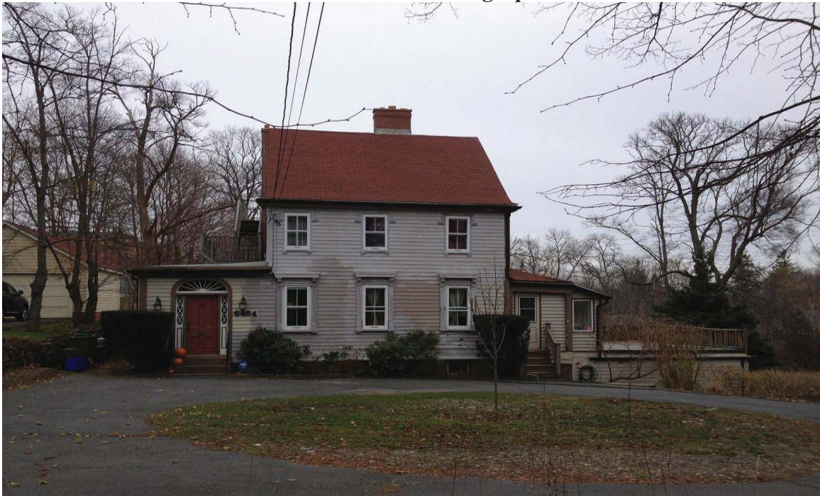
Photograph 1: Front elevation of 6454 Coburg Road, Halifax
