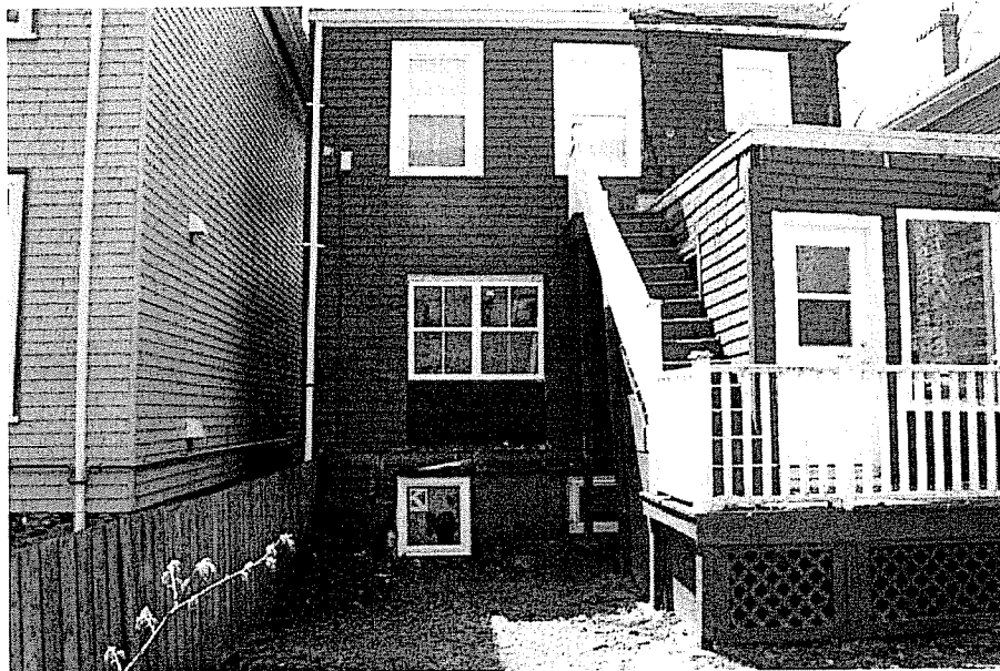
Rear elevation of 1483 Carlton Street showing a new basement window, windows replacing a double door, replaced roof and area on the second floor where a small rear addition was removed.
