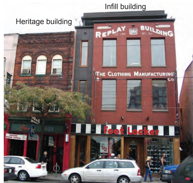
New building in an infill context. Cornice height similarity. Grade height similarity including window proportion and recessed door. Window proportion similarity. Material similarity. Upper storey setback. Stone inset and lettering enhance façade
