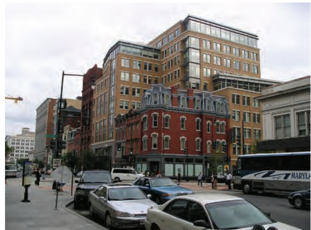
New building negotiates several cornice lines and datum lines between multiple existing heritage buildings. Upper level setbacks. Rhythm similarity. Material similarity. Window proportion similarity.
