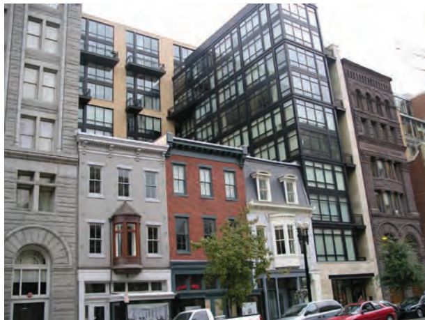
New, larger building setback from heritage buildings. A portion of this new building (black) comes to street edge, where it maintains street rhythm and grade level height. Slight setback at street edge of upper levels. Window proportion similarity. Material contrast
