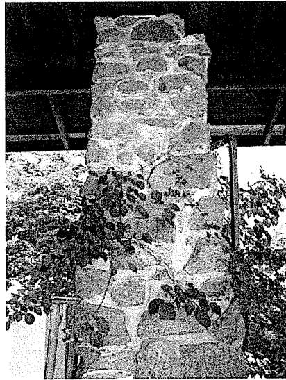
Main house - porch column.
