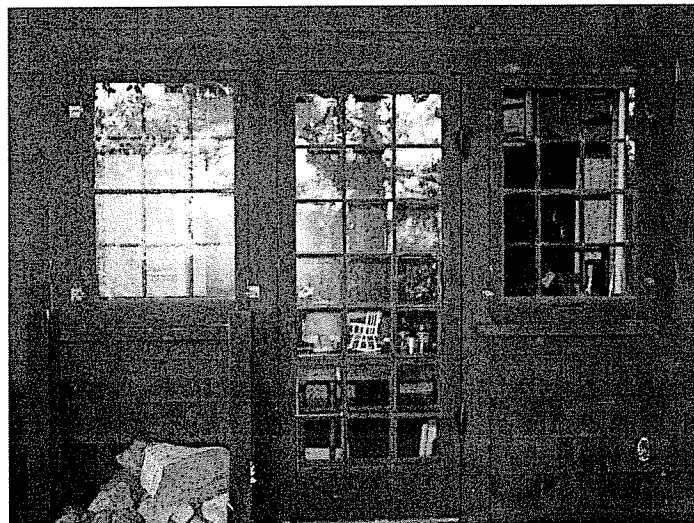
Main house - secondary entrance on front elevation.
