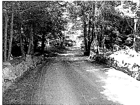
2' dry stone walls lining the driveway entrance (from Kirk Road).
