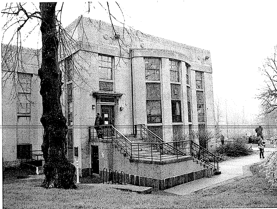
2 Side of building as viewed from Brunswick Street.
