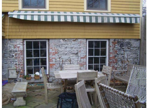
Figure 2: Two ground floor windows at the rear to be removed (2012)
