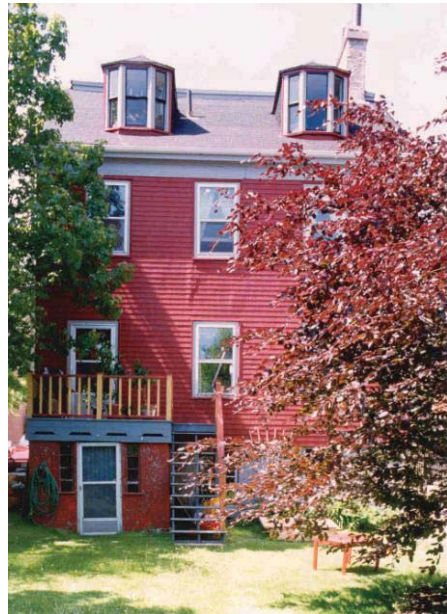
Figure 4: Enclosed rear doorway that was removed (2004)
