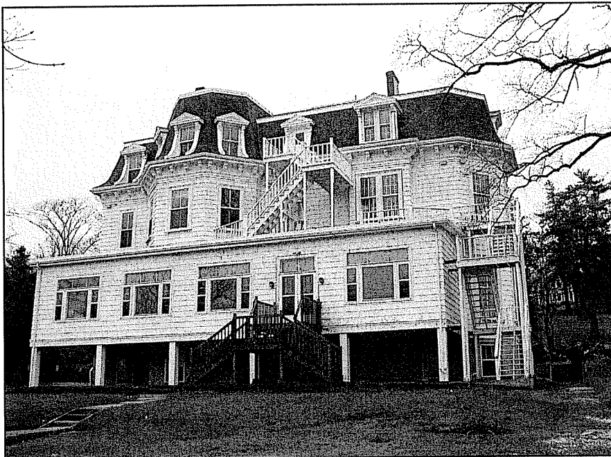
Rear, or waterside, elevation of 1390 Thornvale Avenue.
