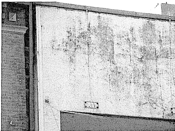
Cracked parging and broken trim on the parapet Exposed holes from old signs allow water penetration.
