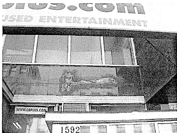
Some original Vitrolite remains in the recessed entry; some is missing; some is painted over.
