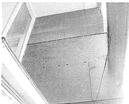
Some original Vitrolite remains in the recessed entry; some is missing; some is painted over.
