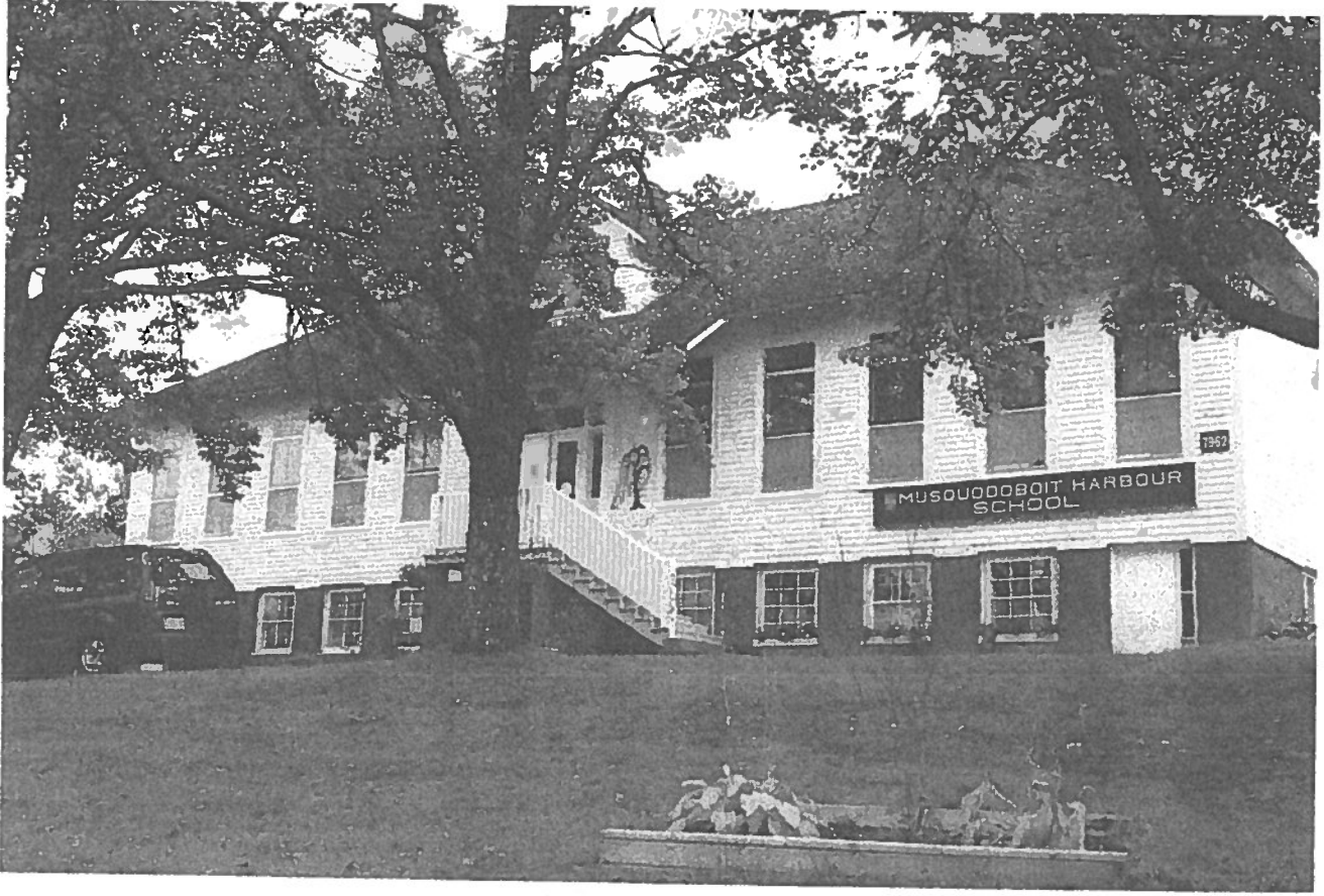
Front elevation of the school building (photo by Colette Bishop-Greene, 2012).
