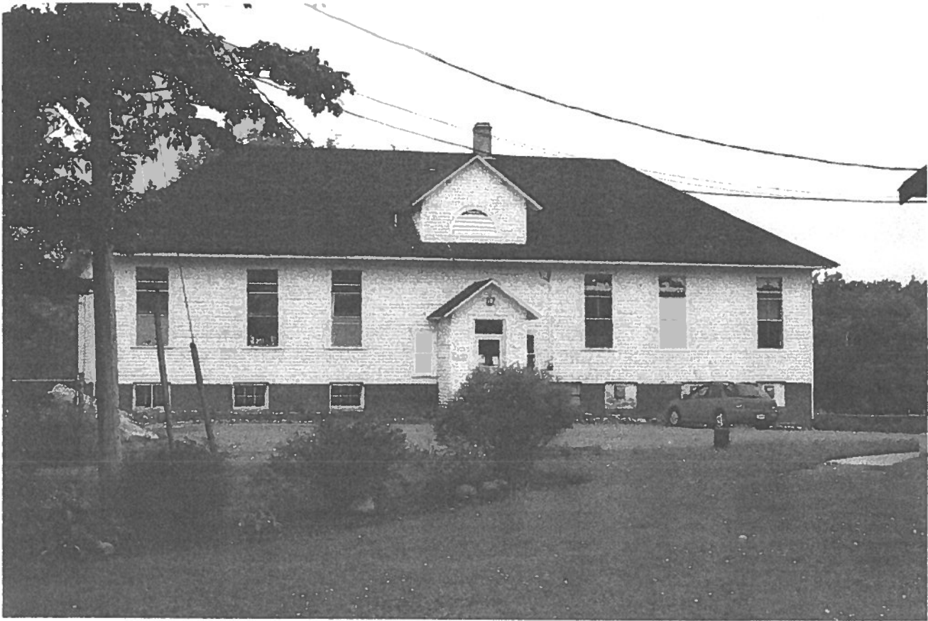
Rear elevation of the school building (photo by Colette Bishop-Greene, 2012).
