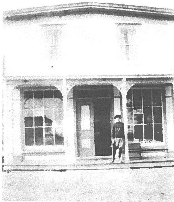
Hosking General Store built in 1896, now located at Memory Lane Heritage Village (courtesy of Eastern Shore Archives).
