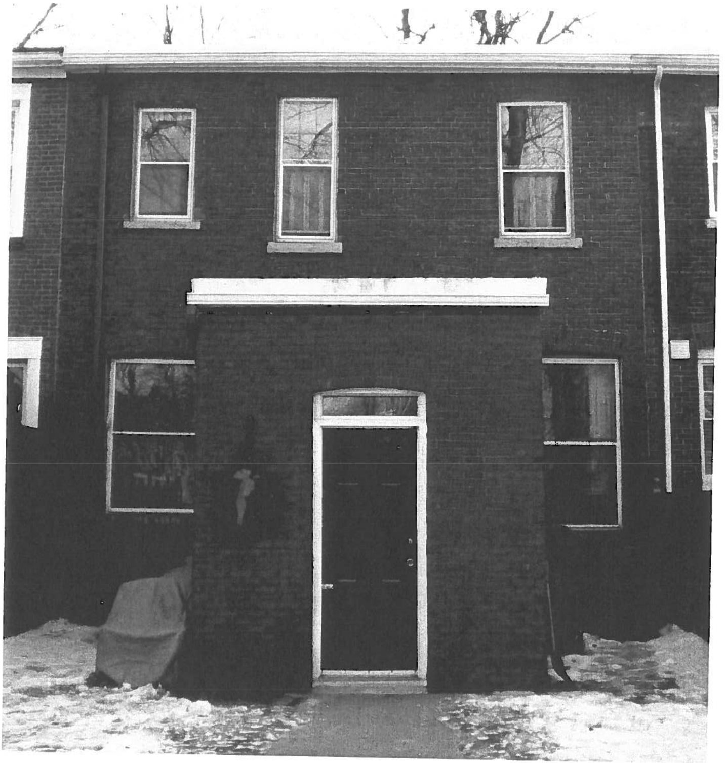
6053 Jubilee Road Rear View
