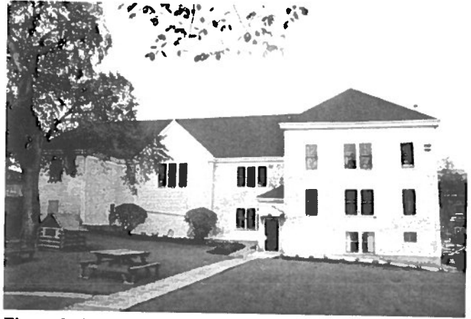
Figure 2: South Elevation – the small existing addition with hip roof currently used as a side entryway is not considered to be a character-defining element
