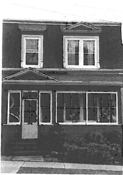
Figure 1: Existing image of the front of the building (T. Kramers)
