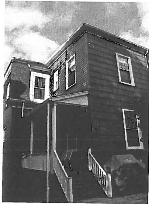
Figure 2: Existing image of the rear side of the building (T. Kramers)
