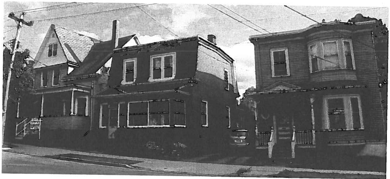
Figure 2: Existing image of the streetscape (T. Kramers)
