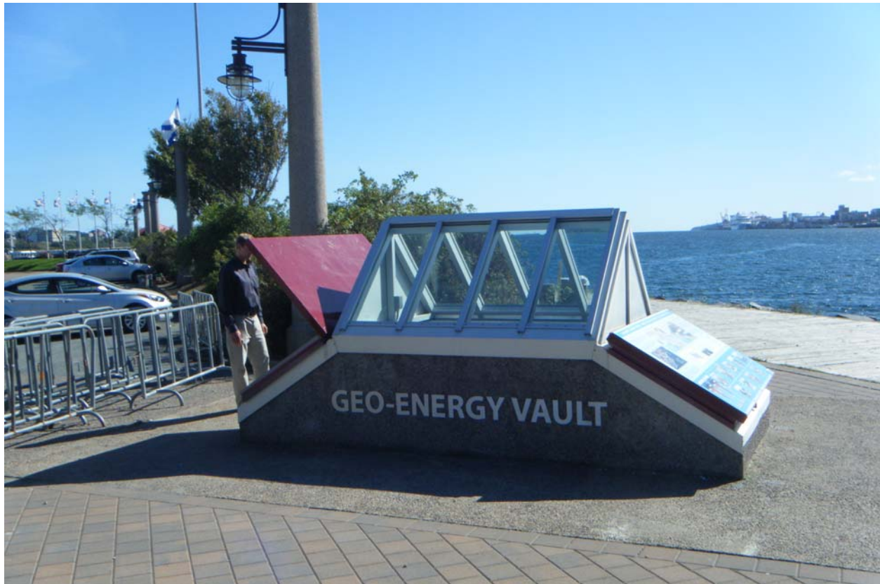
Geo-Energy Vault for Alderney 5 on the Dartmouth waterfront.
