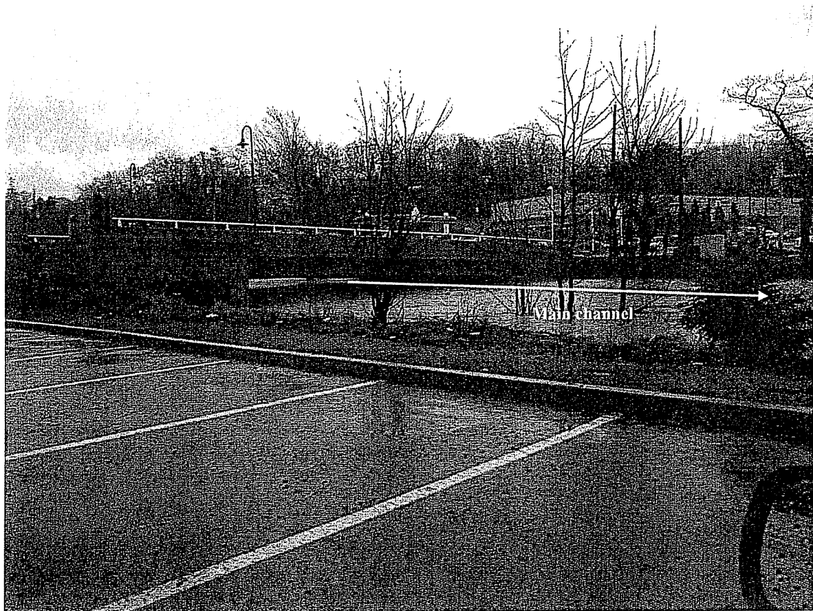
(Downstream Side of 2002 Bridge)
