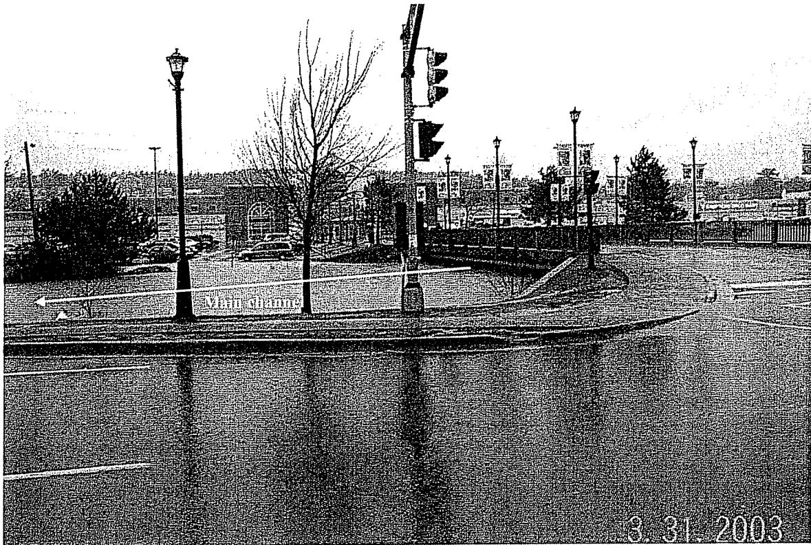
(Downstream Side of Towers Bridge)
