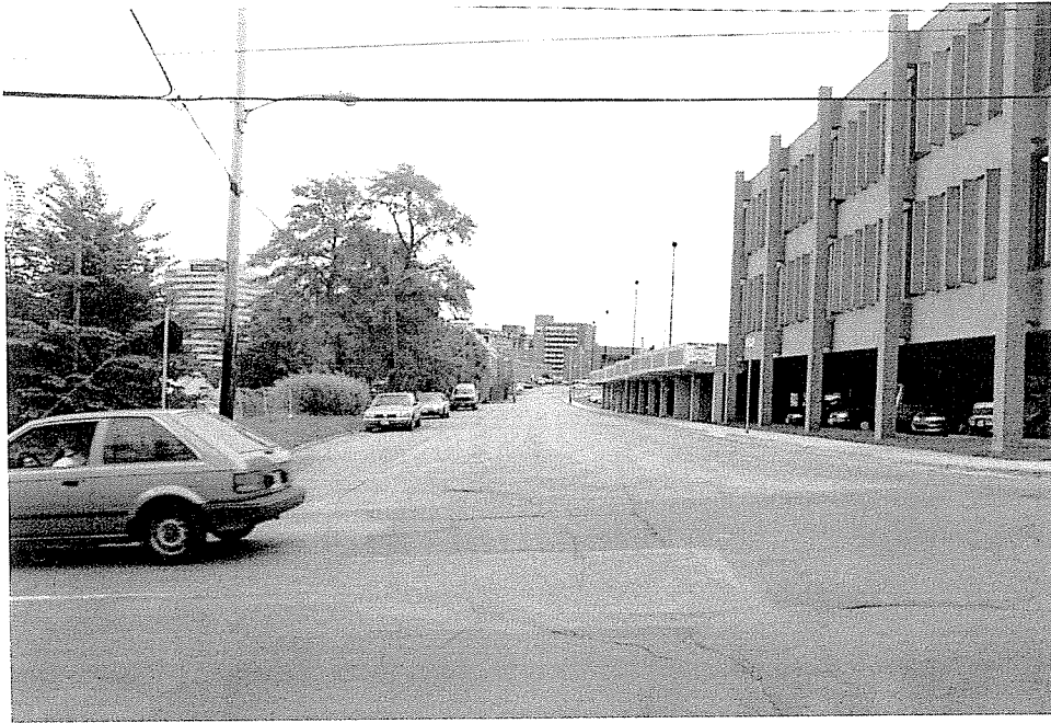
Maitland Street Looking South
