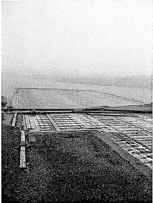
Photo 6: Missing Roofing
