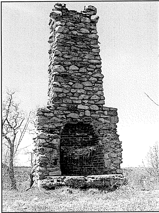
Figure 5: Front view of chimney.
