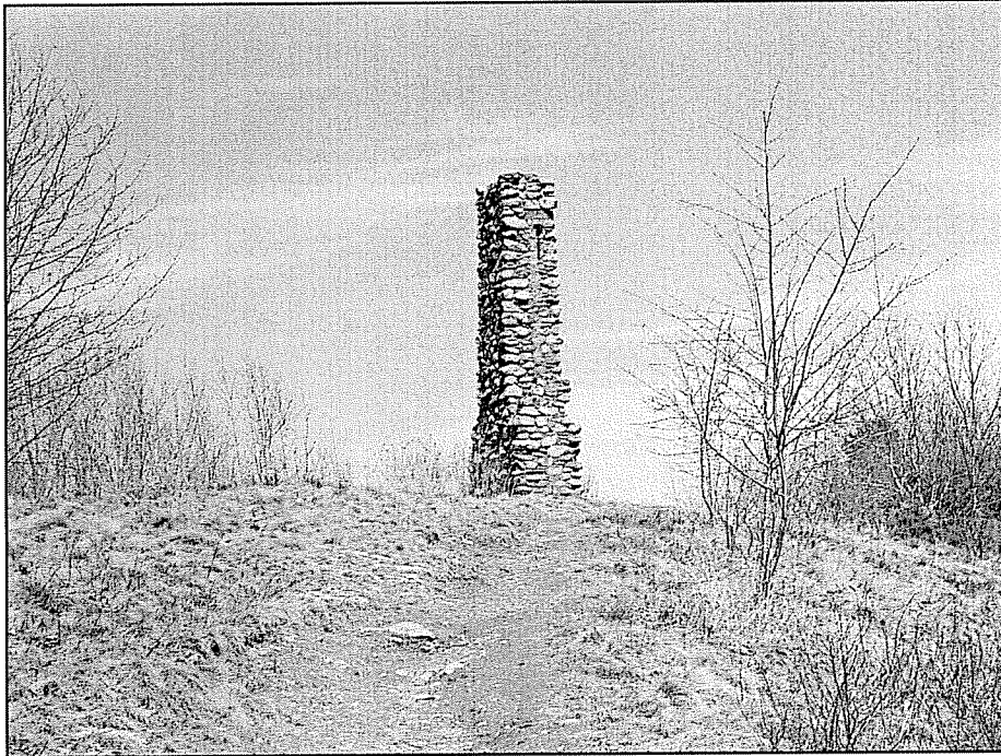
Figure 4: View from the footpath to the Chimney.
