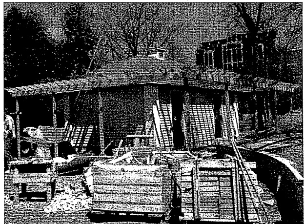
New Men's and Family Washroom
