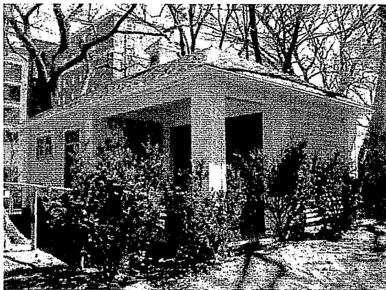
New Maintenance Shed
