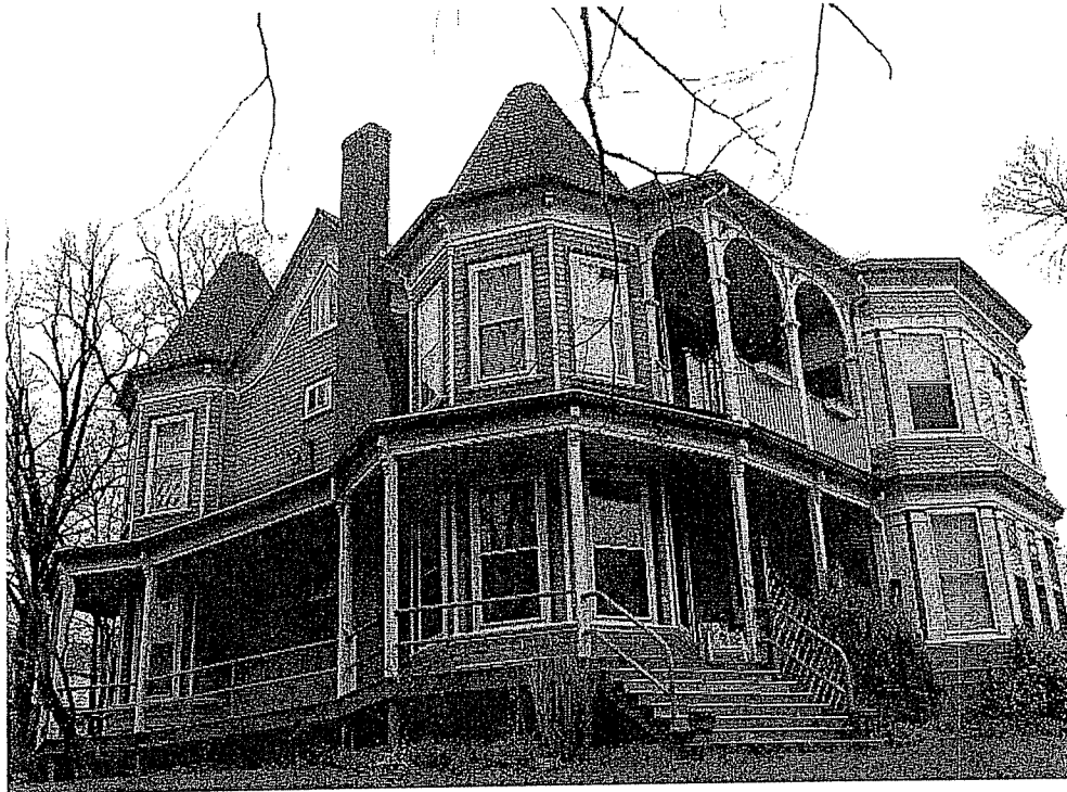
1991 Prince Arthur Street (Pinehurst), Halifax.
