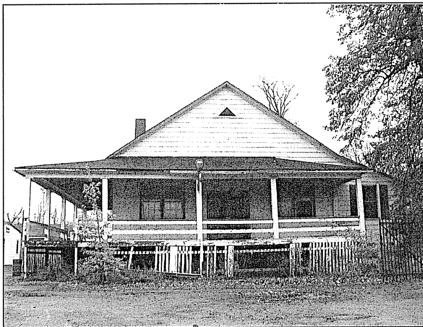
West facing elevation of the Dry Canteen.
