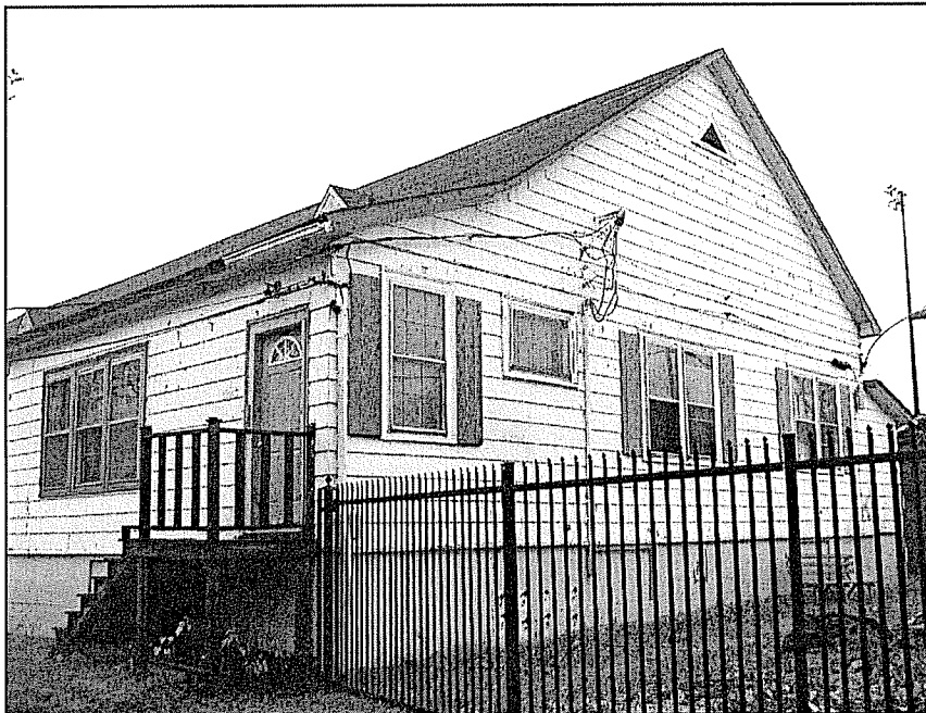
East facing elevation of the Dry Canteen.
