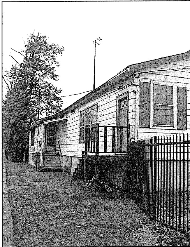
View down the South facing elevation (Sackville St).
