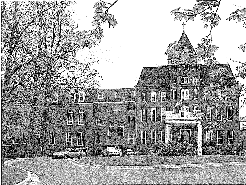
Historic Elements: 1851 Main Building and 1876 East Wing
