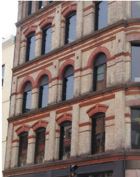
Yellow and red brick with terra cotta accents on cornices, string courses and window heads
