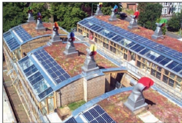
Green roofs, natural ventilation and solar panels
