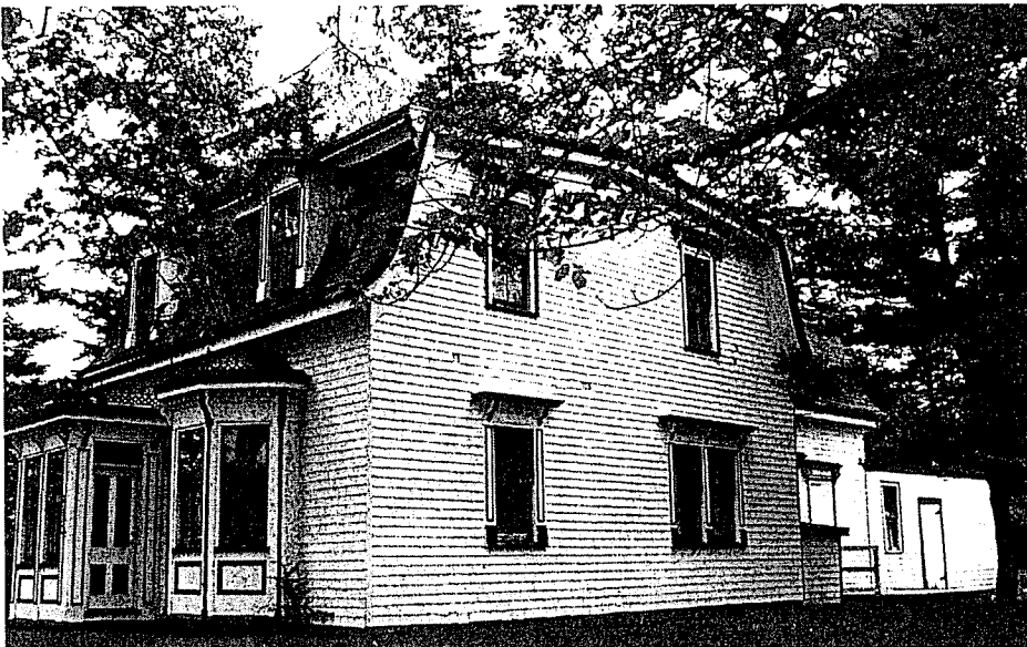
North west elevation: single and double windows with hood mouldings. The photo also shows the rear addition.
