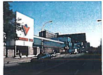
The blank wall along Quinpool Centre creates an uninviting environment
