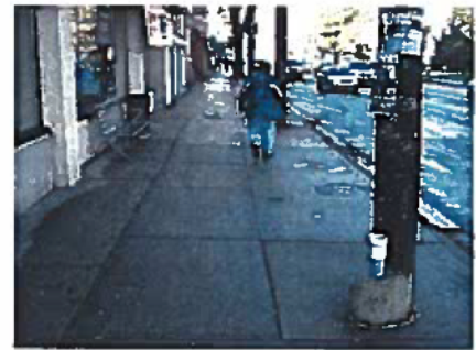
The existing sidewalk width on Quinpool Road between Robie and Vernon Street
