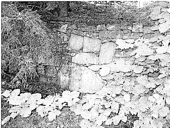
5' high dry stone wall (near main house).
