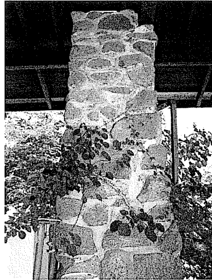
Main house - porch column.
