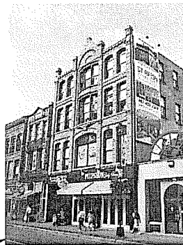
1717 Barrington G.M. Smith Building
