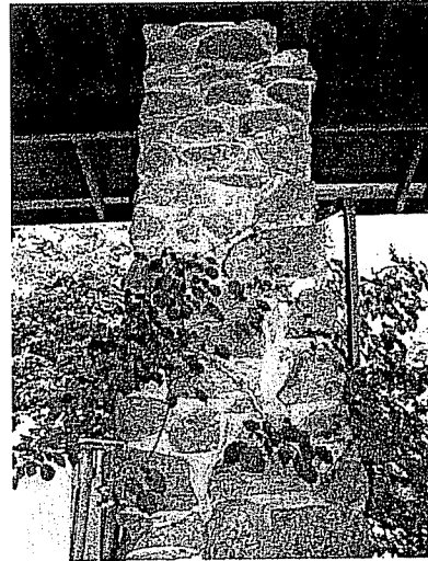
Main house - porch column.
