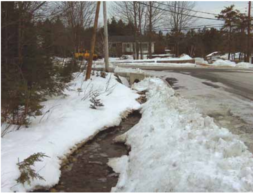
Fenerty Road storm sewer system
