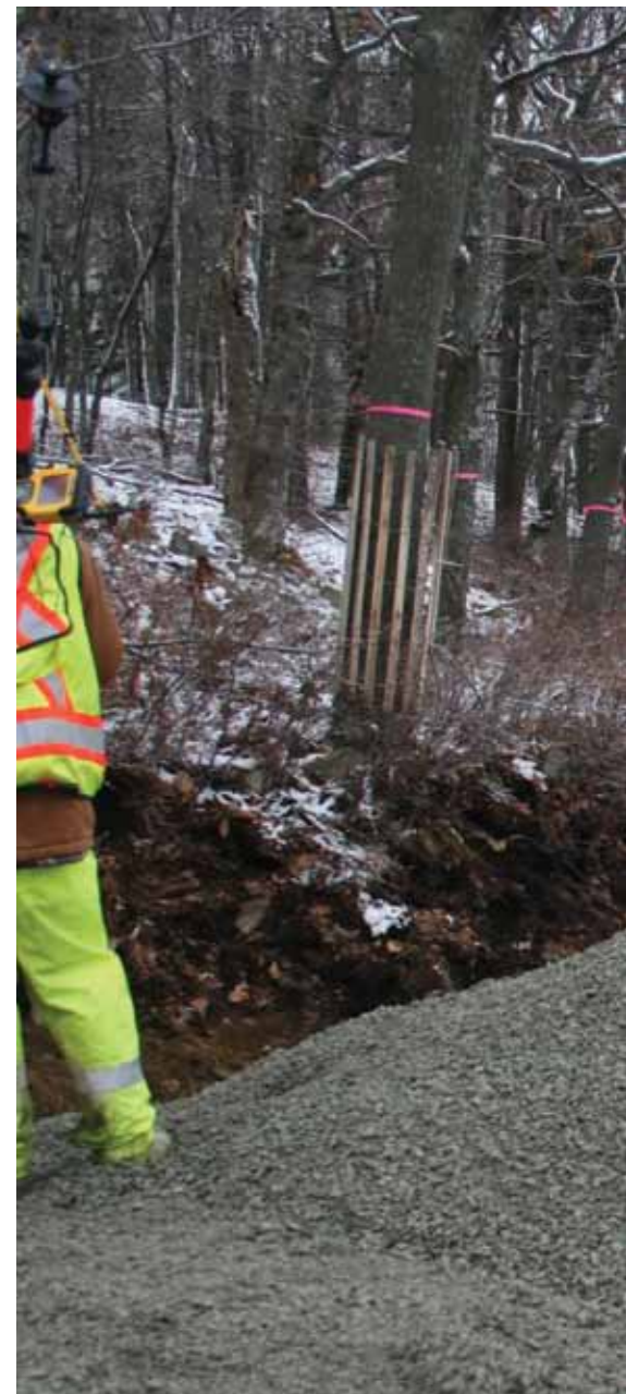
Below: North Dartmouth Trunk sewer project
