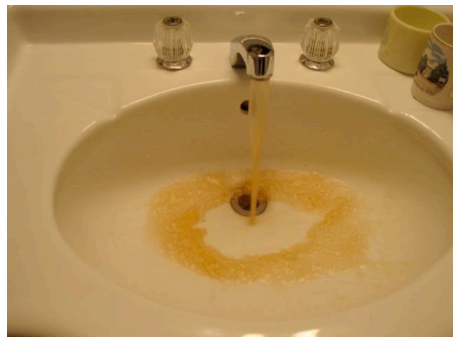
Figure 7 - Discoloured water, after running a minute, Sept.10/09
