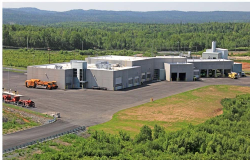
Combined Services Complex
