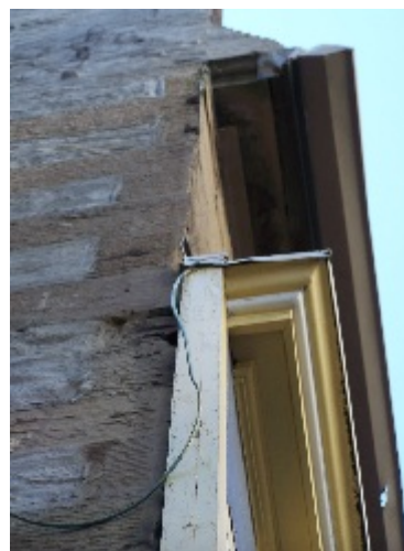
Gaps between masonry corners and storefront trim
