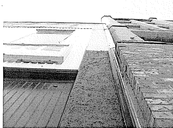
Broken trim on second floor window. Mismatched corner trim over parging.
