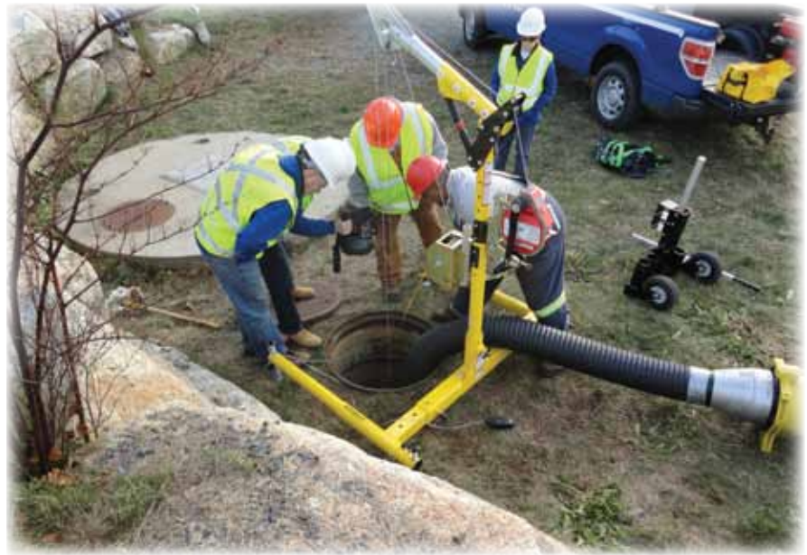
Confined space entry using proper tools and procedures
