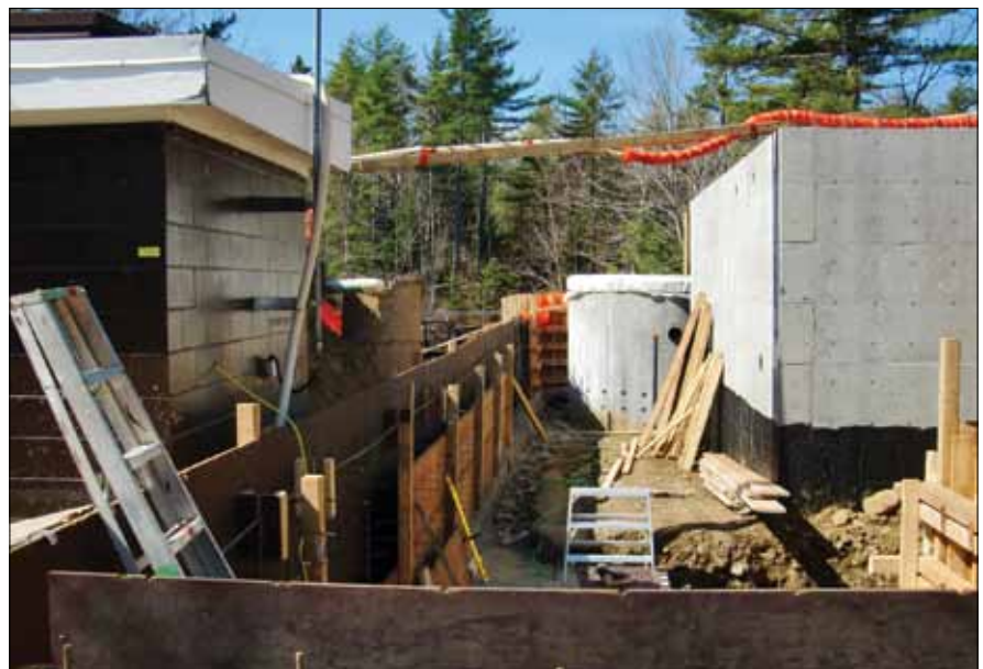
New Wellington WWTF being constructed to improve effluent quality
