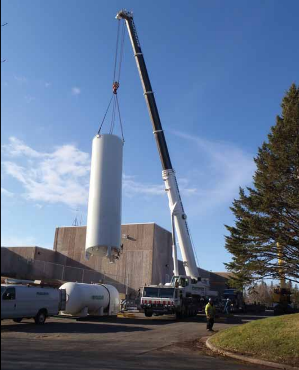
JD Kline Water Supply Plant receives a new Carbon Dioxide tank
