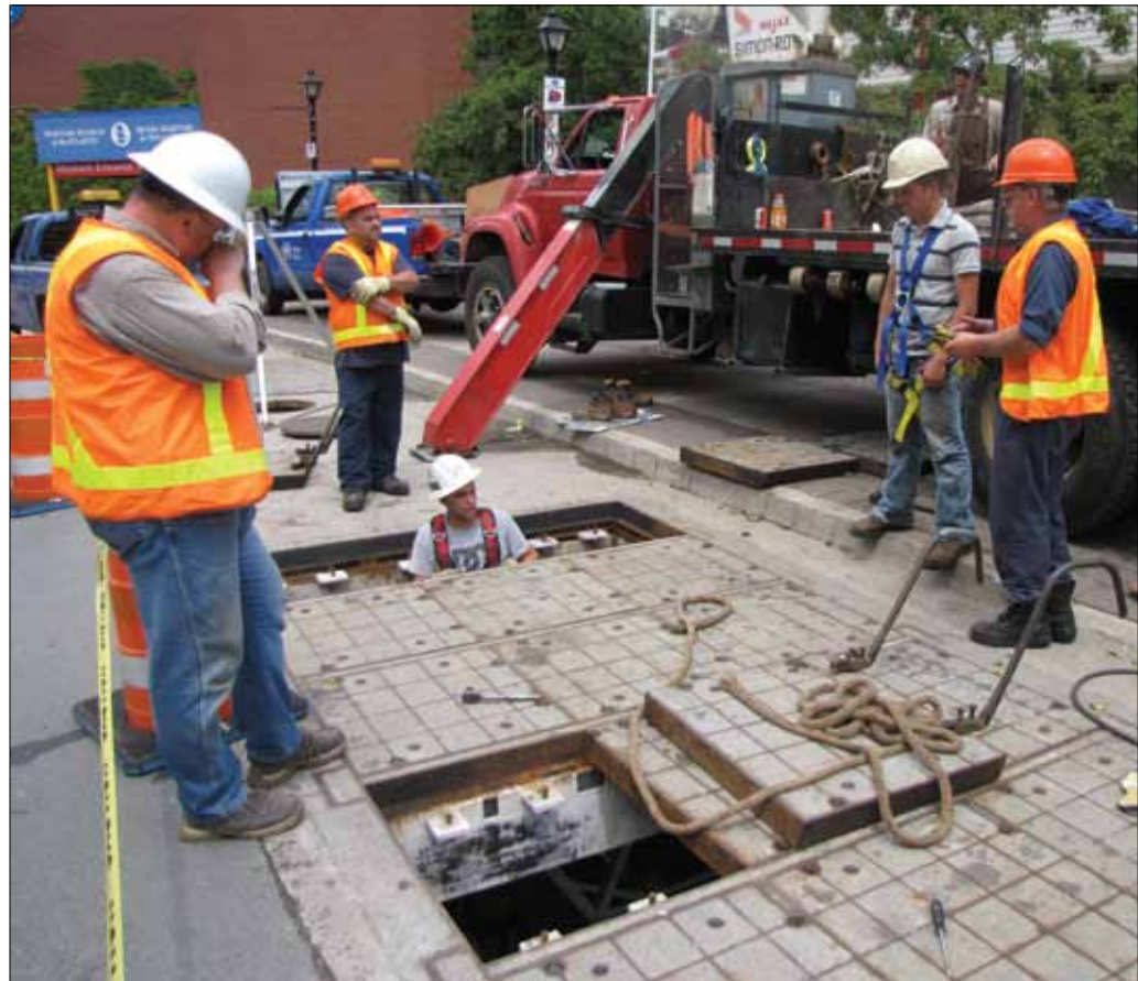
Workers maintain wastewater system along Lower Water Street, Halifax
