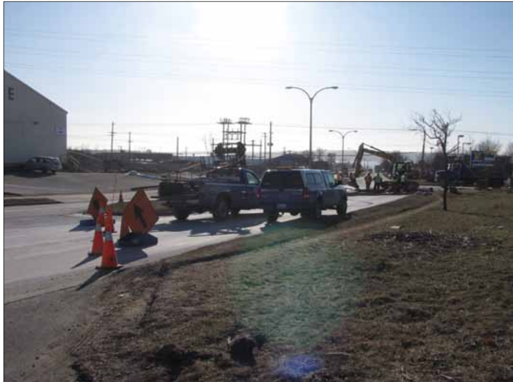
Traffic set up for a safe construction site
