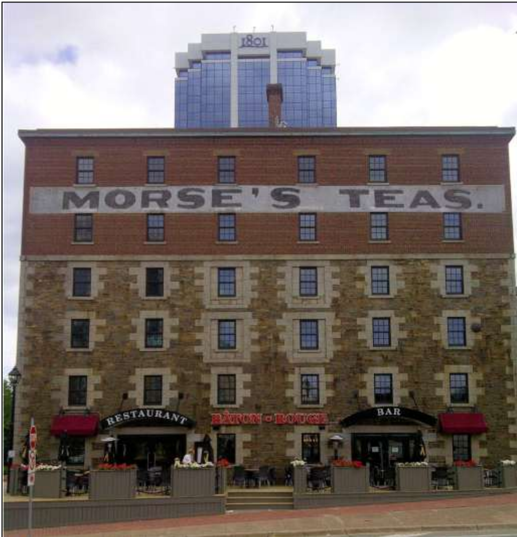
Recent Photograph (2011): Morse's Tea Building, 1877 Hollis Street, Halifax, after renovations to allow the new tenant the Baton Rouge restaurant.
