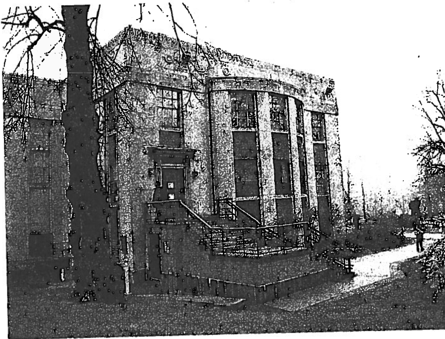
2 Side of building as viewed from Brunswick Street.
