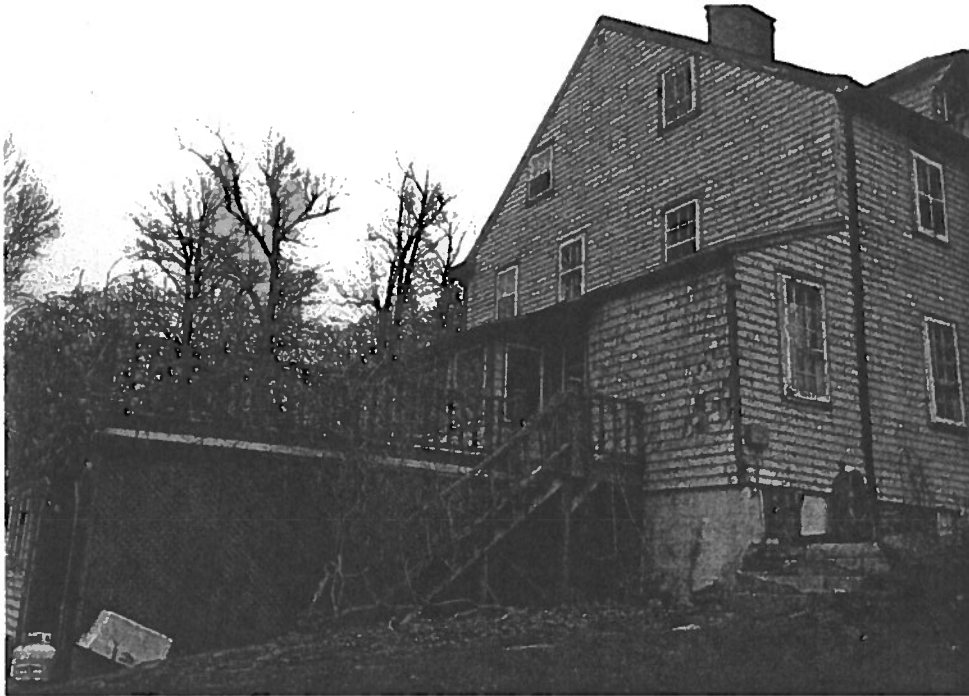
Photograph 3: Rear view of sunroom and carport
