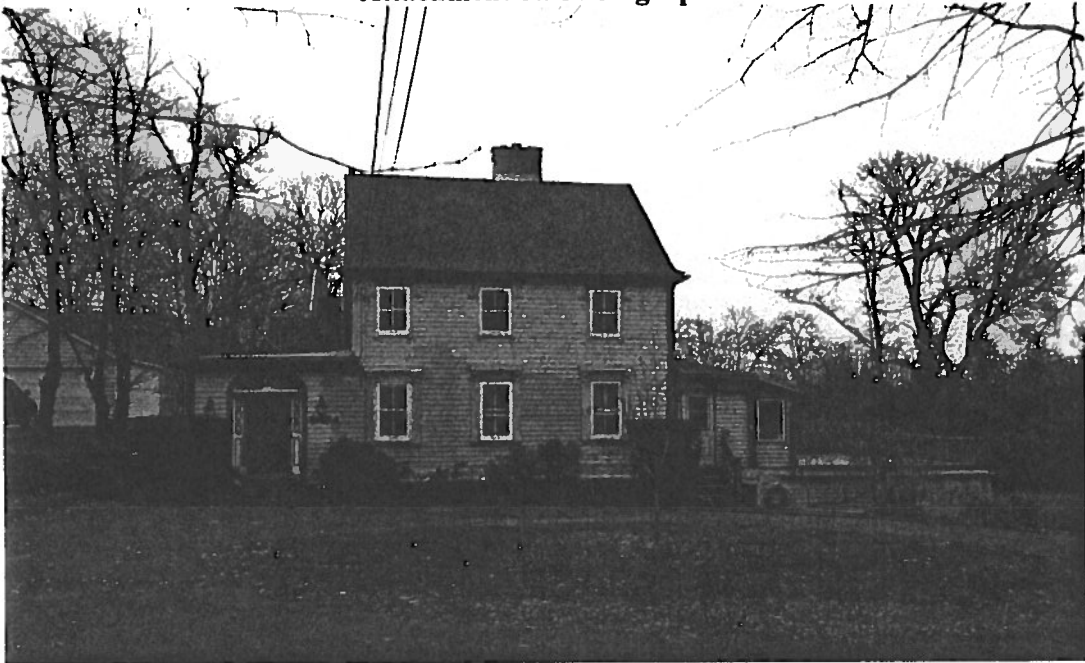
Photograph 1: Front elevation of 6454 Coburg Road, Halifax
