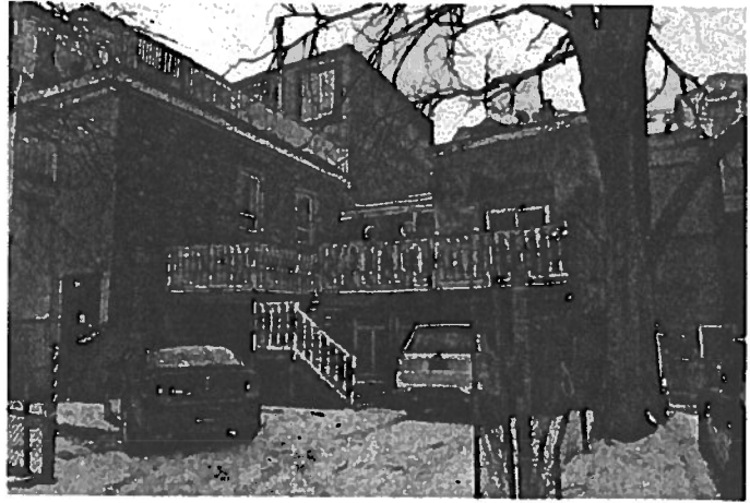
Figure 2: Existing rear addition and deck from 1988 to be removed
