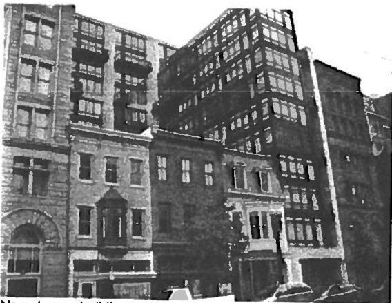
New, larger building setback from heritage buildings. A portion of this new building (black) comes to street edge where it maintains street rhythm and grade level height. Slight setback at street edge of upper levels. Window proportion similarity. Material contrast
