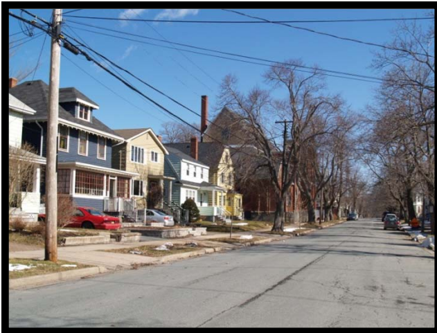
Along Willow Street, facing east – church building and yellow house are the subject site
