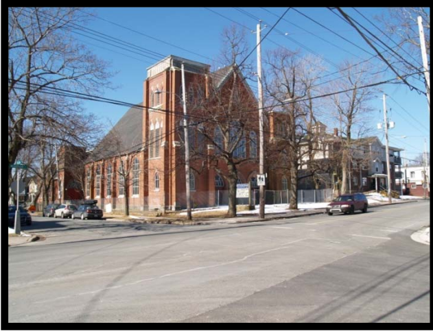
South-east corner of the church building; front facing Windsor Street
