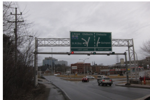
Armdale Roundabout at Herring Cove Road
